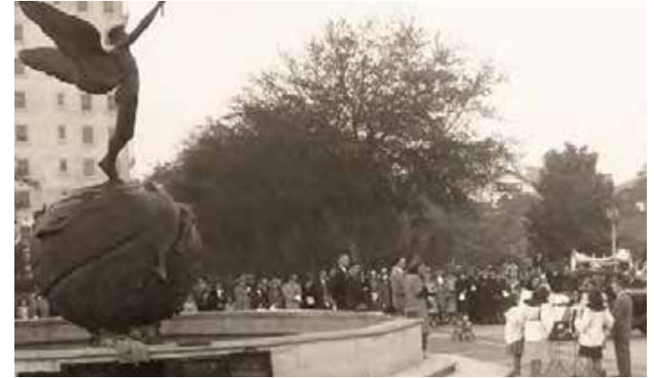
Enlargement of previous picture showing a spotlight (far right) installed on a pole for illuminating the sculpture.
