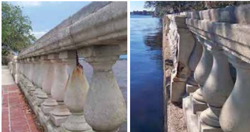
Above, original design detail of balustrade (courtesy Olmsted NHS) and circa 1949 appearance (courtesy JHS); below, current profile with added cap layer. Note also exposed, rusting reinforcing steel.
