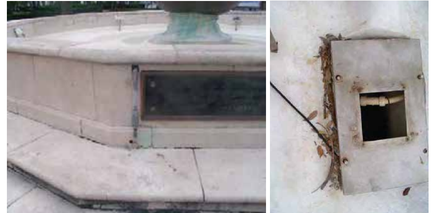
Old electrical work mars some of the fountain's cast stone cladding (left); the current pump vault is undersized and the pump out of commission (right). Fountain restoration must address plumbing systems, controls, the basin lining and full restoration / repair of all of the cast stone work.
