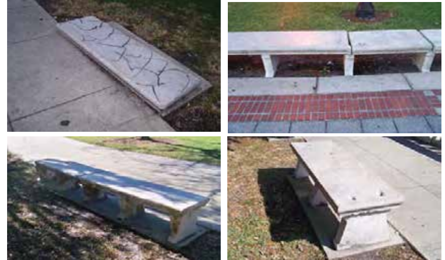
Benches also suffer from graffiti, breakage, discoloration, occasional spalling and other wear and tear.
