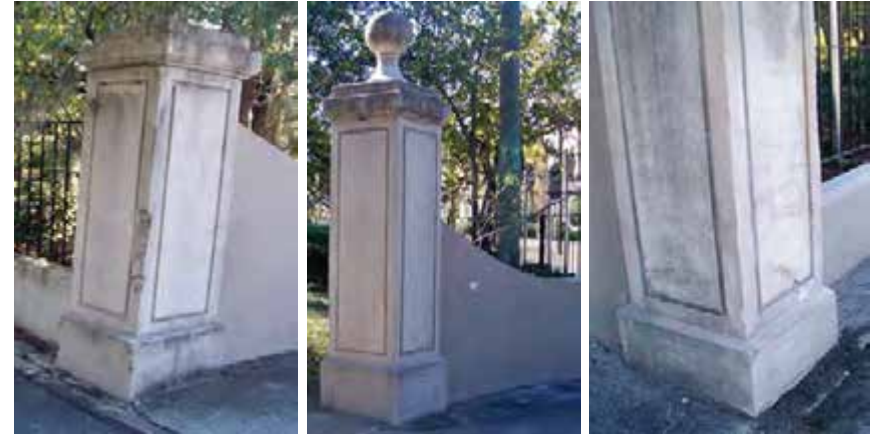
Northeast entry (left to right): damaged pier; peeling paint; damaged pier.
