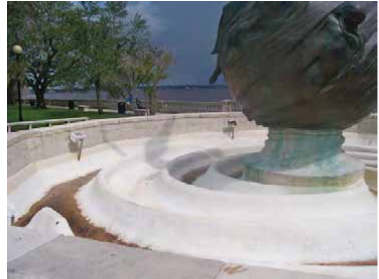
The installation of lights and electrical conduit in the fountain basin wall has damaged the interior surface and is visually intrusive.
