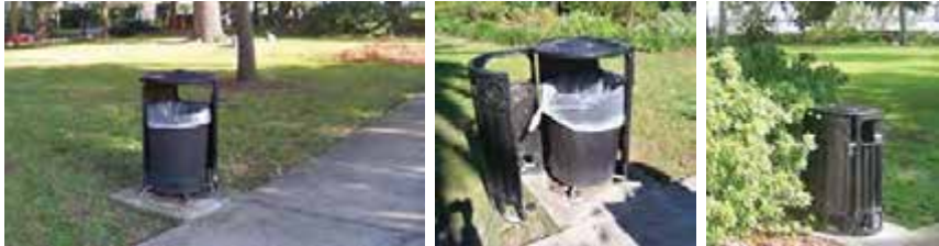
The existing receptacles were installed in 1994. Several no longer stay reliably closed or are missing the side door panel.
